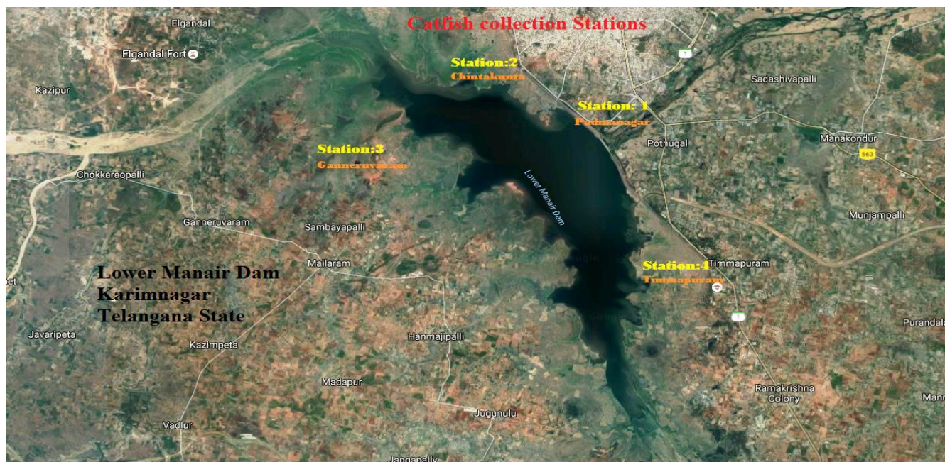
Fig. 1: Lower Manair Dam
